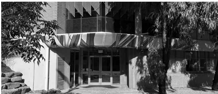
Front door to the newly refurbished Moondani Balluk Centre.
